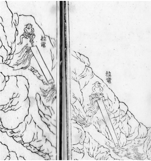
FIGURE 6. Miners using two layers of water pumps for water drainage. The water drainage methods described in Wu Qijun's mining treatise were more closely aligned with an illustration found in Japanese copper mining records (see fig. 7). Detail from Wu Qijun, An Illustrated Strategy of Mining and Smelting Tools in Yunnan (1844). Woodblock print, 30.5 × 20.5 cm. Courtesy of Nanjing Library, China.
